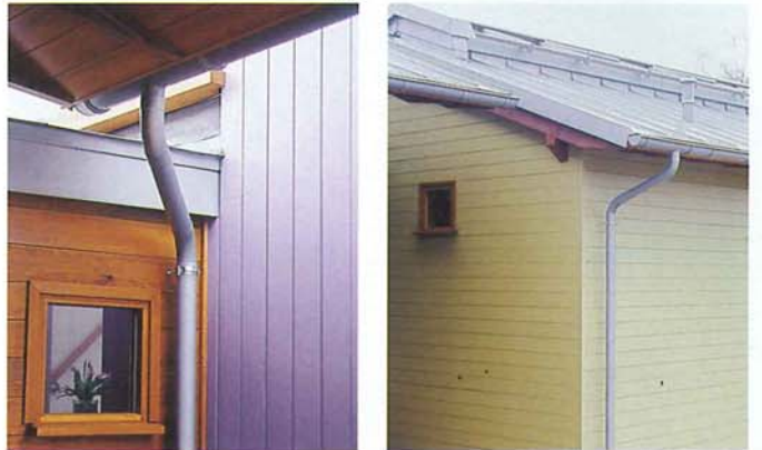
5. Purple and green paint on exterior wood by Sikks
